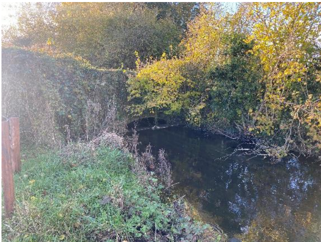
Plate 5: Arch of road bridge CH1.
